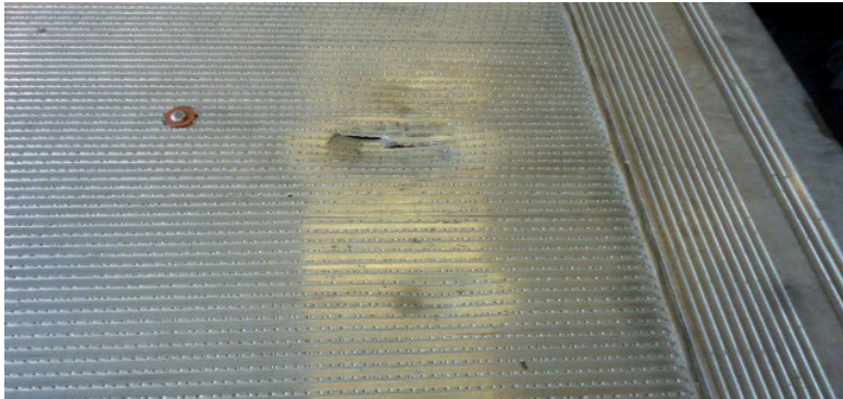
✘ Cargo liftgate/impact damage • Material deformations, fractures
